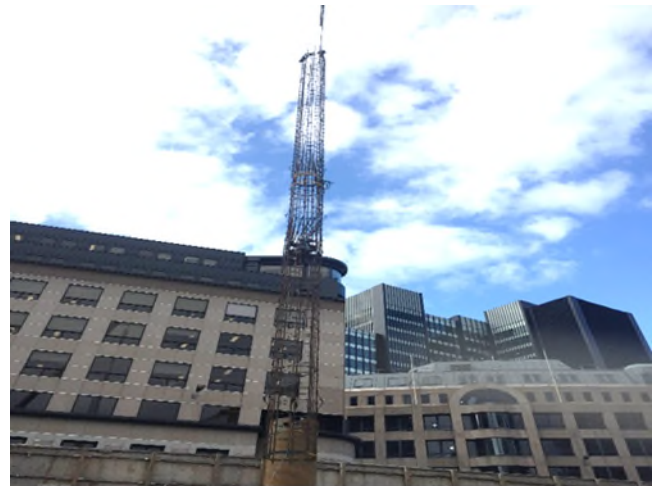
Installation of the reinforcing cage and instrumentation into the pile
