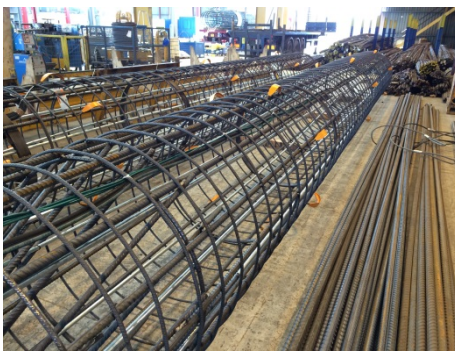
O-cell assembly made at AMCS's cage fabrication facility in Kent.
