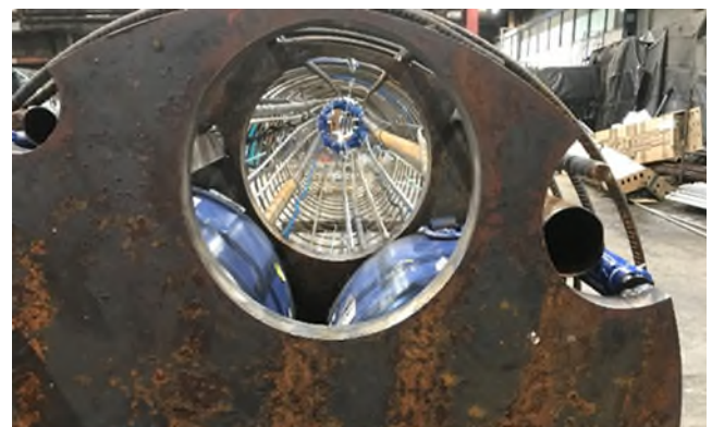
Reinforcement with O-Cell® assembly ready for installation
