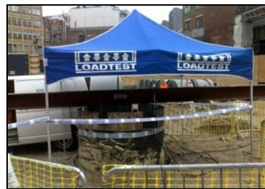
Testing in progress – pile head and reference beam
