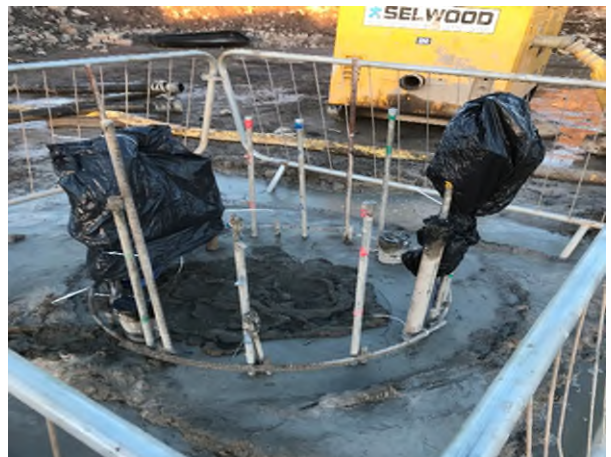
O-Cell® test installed and concreted
