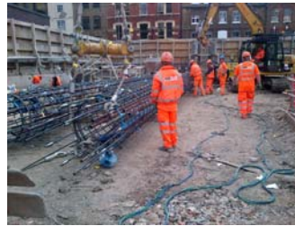
Instrumented cages ready for lifting
