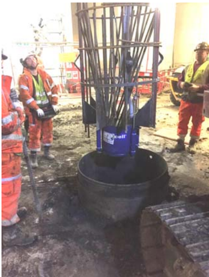
Installation of the O-cell and reinforcing cage for the test pile
