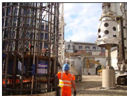
Installation of one of the preliminary test piles
