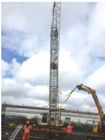
Installation of one of the working test piles
