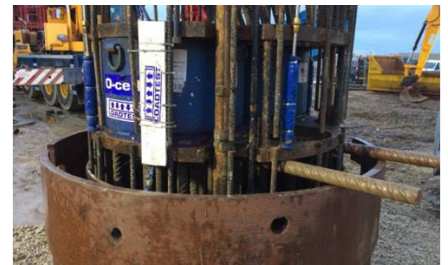
Installation of one of the preliminary test piles
