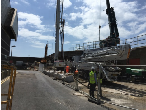
Photographs showing the congestion in the site
