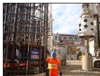
Installation of one of the preliminary test piles
