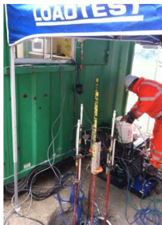
Pile test at C123 in progress
