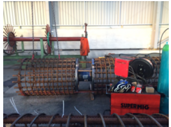
O-cell assembly made at the cage fabrication facility
