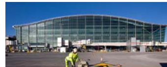
The Completed T5 Building at Heathrow
