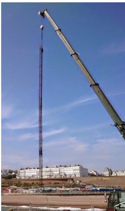
Lifting of full length reinforcing cage .
