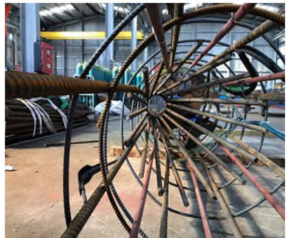
Reinforcement with O-Cell® assembly ready for installation
