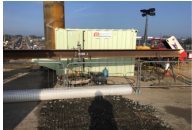
Testing in progress – pile head and reference beam
