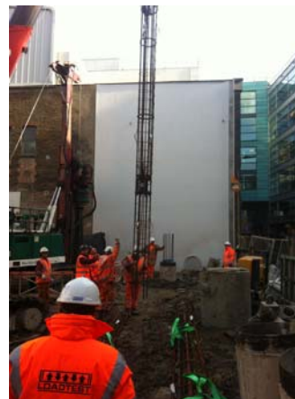
Single O-cell cage installation
