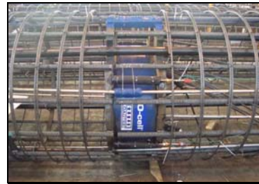
O-cell assembly made at Rom-Tech's cage fabrication facility in Sheffield
