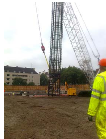
Lifting of the pile cage with O-cell assembly
