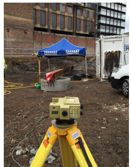
Testing in progress – monitoring pile head movement.
