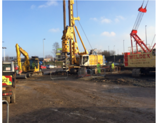
Installation of one of the working test piles
