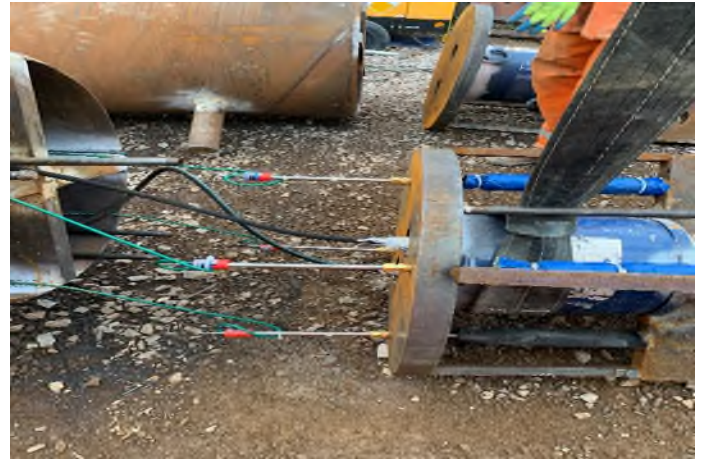
Installation of O-Cell® assembly and its instrumentation into the pipe pile
