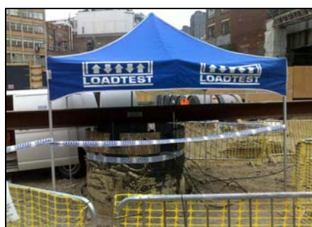
Testing in progress - pile head and reference beam
