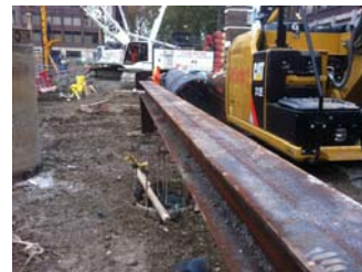
Test pile prior to testing
